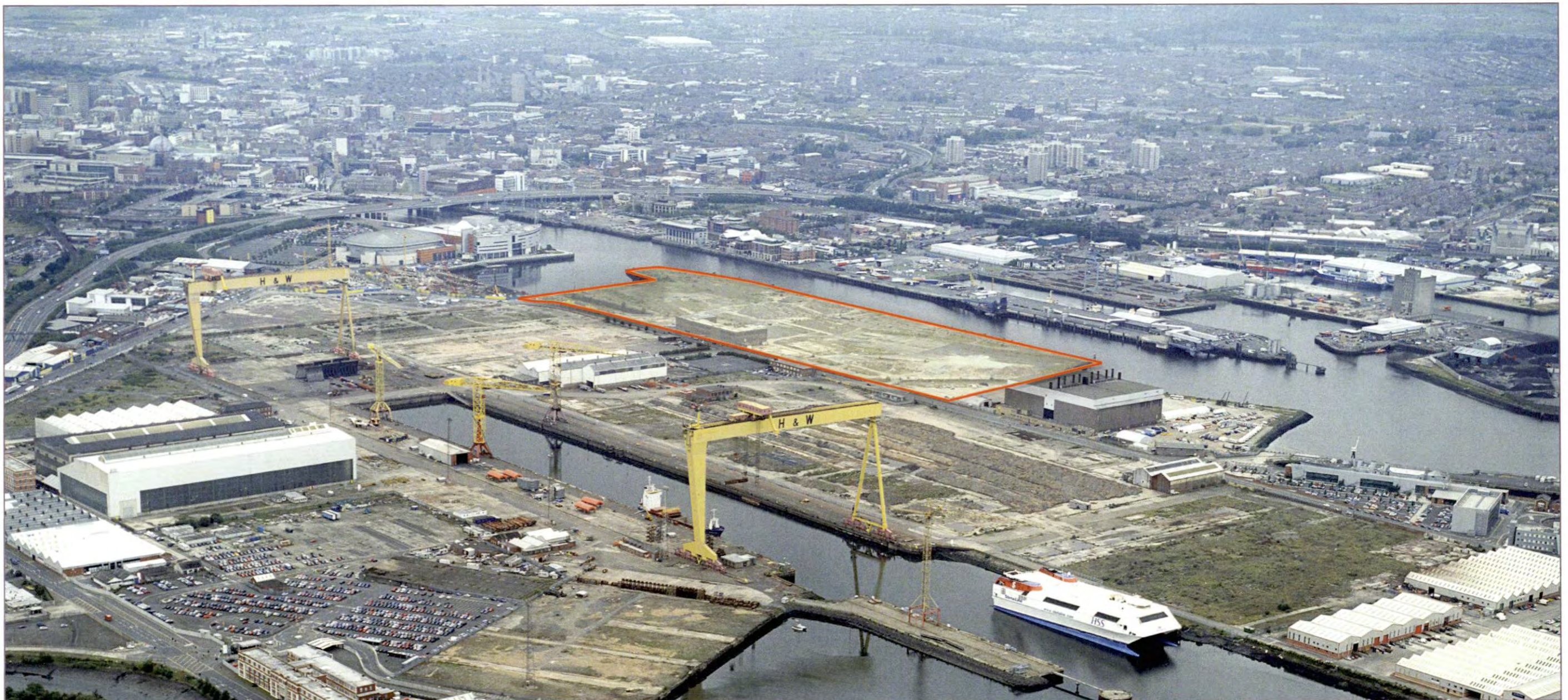
Fig 1.3 Aerial view of the Titanic Quarter Phase II
